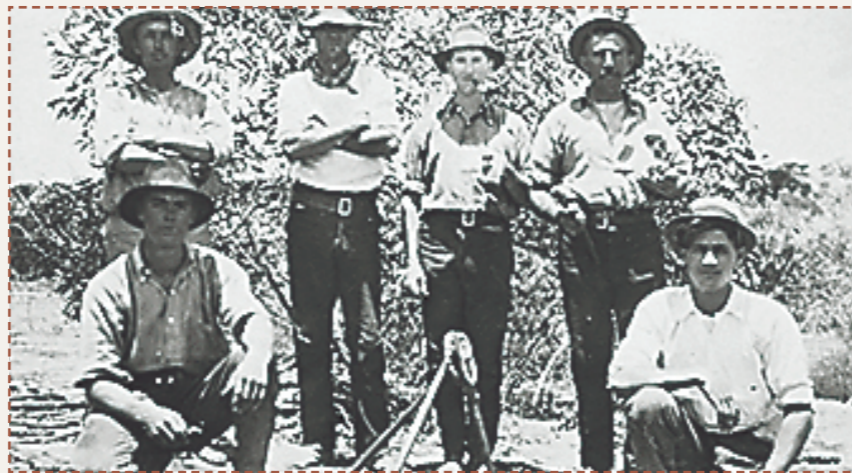
Workers on the Trans-Australian Railway, about 1915. The construction of the 1 693 km line took about five years. National Museum of Australia.
